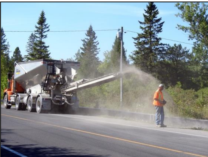
Back-filling fence with gravel
