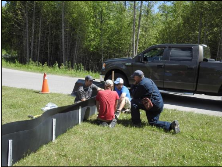
Team install wildlife fencing near Park Store
