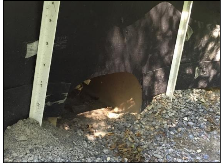
Wildlife tunnel positioned in the fencing encourages wildlife to use safe crossings
